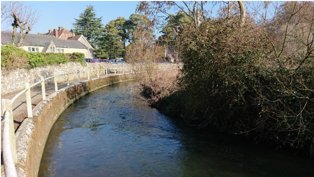
Figure 3: Natural riffles towards the end of the reach visited. This figure also shows the concrete revetment.
